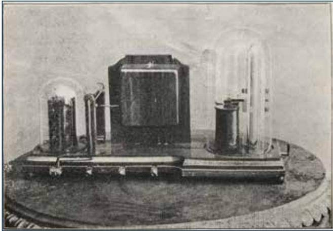
Fig. 11 This Boggio-Lera lightning detector (without recording device) was installed in the Royal School of viticulture and oenology of Catania. From left to right: lightning protector; metallic powder coherer; electric de-cohering hammer and Hipp's relay. (Boggio-Lera, 1901, op. cit. note 34).
